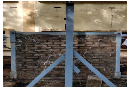
Figure 14. Experimental Crack Pattern After Cyclic Loading.
