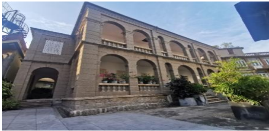
Figure 9: Private Kulangsu Hospital (1925, Kulangsu)
