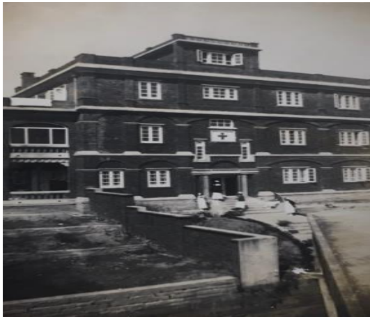
Figure 14: The nursing school of Hope Hospital
