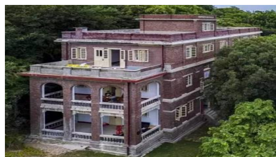
Figure 8: Hope Hospital (1898, Kulangsu)
